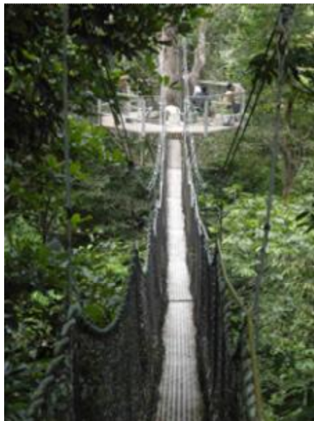
Atta Canopy Walkway – Chris Collins
